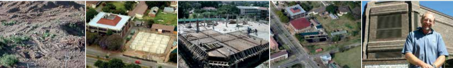
The Collections building taking shape, and the completed facility in 2007.
