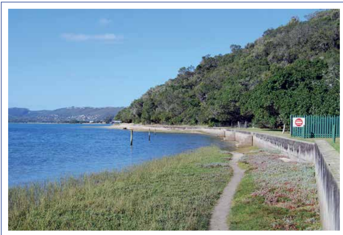
Figure 4.19 Shoreline armoring to protect roads and houses and other property changes the composition of the estuary margins and restricts the estuary's natural ability to change shape. These vertical structures at Brenton on Lake have altered the morphology of the shoreline and will lead to loss of the fronting saltmarsh as sea level rises (Photograph: © Alan Whitfield).
