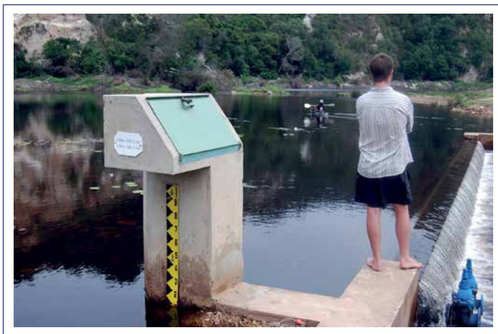
Figure 12.16 This photograph shows the Department of Water Affairs & Sanitation flow gauging weir at the head of the Knysna Estuary. Regular monitoring of Knysna riverine water quality and quantity inputs, together with a range of estuarine ‘health’ indicators, is required for future wise management of the system (Photograph: © Alan Whitfield).
