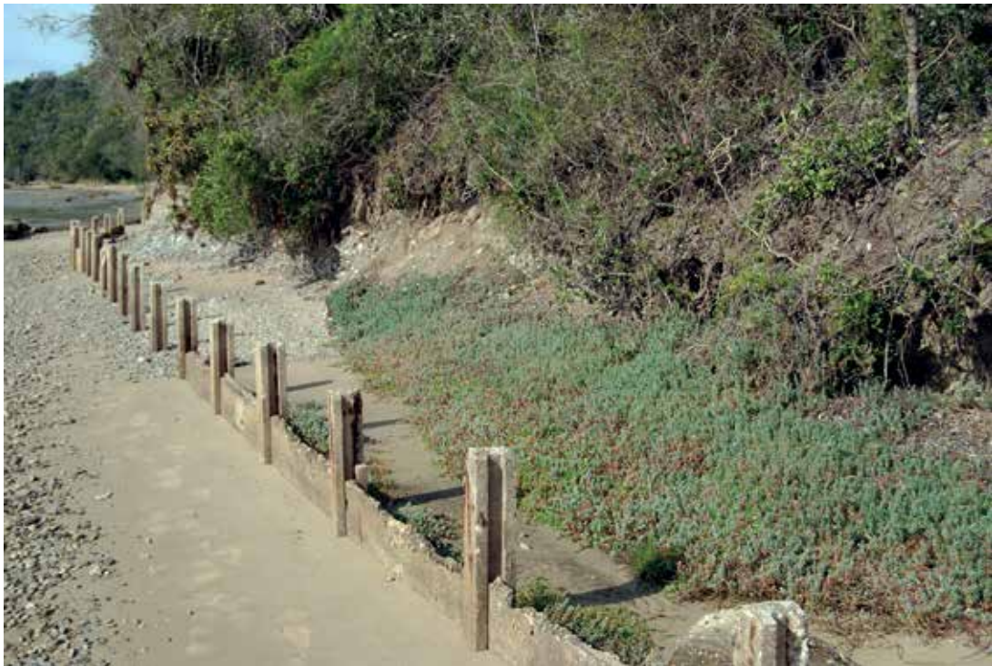
Figure 12.6 A failed attempt to prevent the expansion of the southern shore of the Knysna Estuary using a precast concrete fence structure. Such hard structures in selected areas should be removed to allow the estuary to follow its natural evolutionary path (Photograph: © Alan Whitfield).
