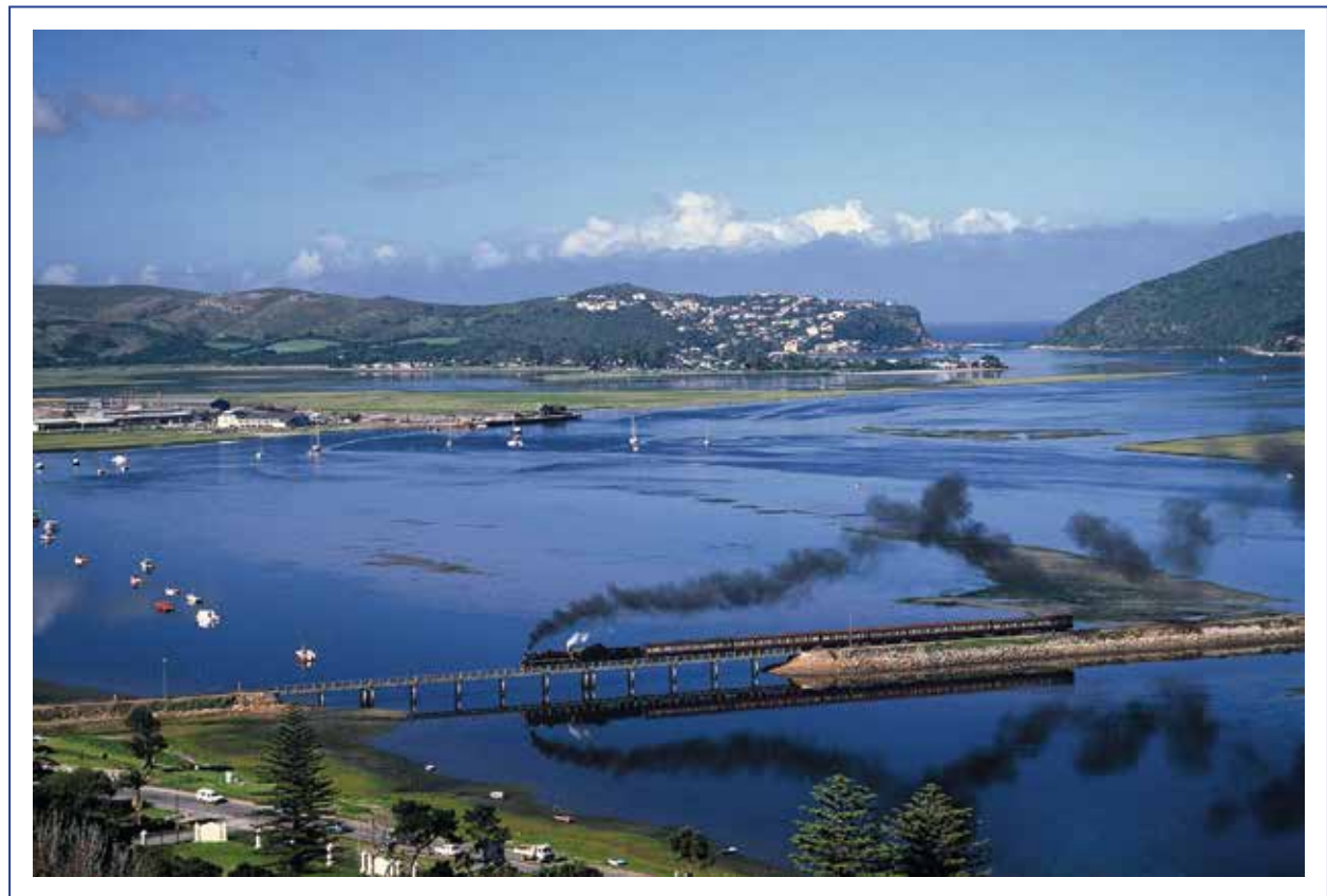
Figure 4.7 Drilling for the railway bridge pylons to 24 m depth failed to reach bedrock of the valley in which the Knysna Estuary is situated (Photograph: © Heinrich Von Horsten).
